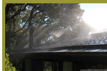
Photo 1. Roof mounted sprinkler.
