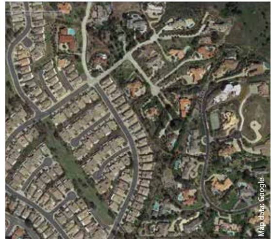
Figure 11. High- versus low-density development north of Poway, California. Tighter clustering of housing decreases amounts of flammable vegetation, which makes defensible space easier to maintain. During a wildfire, high-density development can also be defended more easily and with fewer resources.
