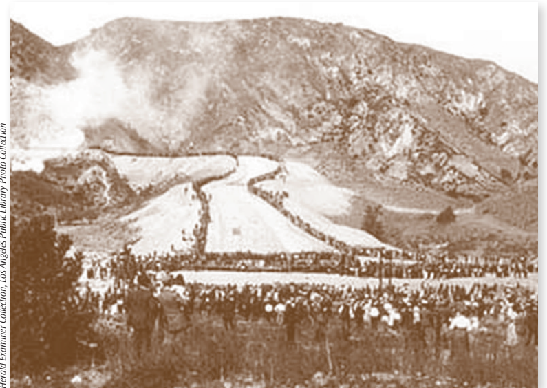
THE LOS ANGELES AQUEDUCT ENTERING THE SAN FERNANDO VALLEY, 1913.
