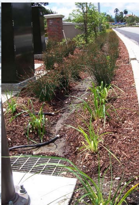
Figure 35. This bioswale was installed during a road widening project in Menlo Park, California, to mitigate for the additional runoff caused by additional impervious surfaces. The swale is constructed with a layer of aggregate under the soil and is planted with wetland species. The curb along the road has gaps to allow water to flow into the swale. A catchment was installed (under the grate) to allow sediment to settle out of the storm water before discharge to the creek. Photo: R. Harris.
