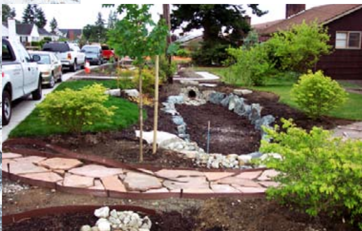
Figure 28. Swales retain rainwater and grow rain gardens to enhance the neighborhood. Source: © 2005, Seattle Public Utilities, used with permission.
