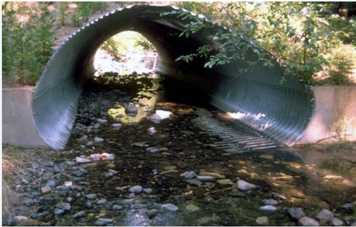
Figure 20. A natural-bottomed arch culvert installed on a fish-bearing stream minimizes impacts on fish habitat and migration. Source: Keller and Sherar 2003, used with permission.
