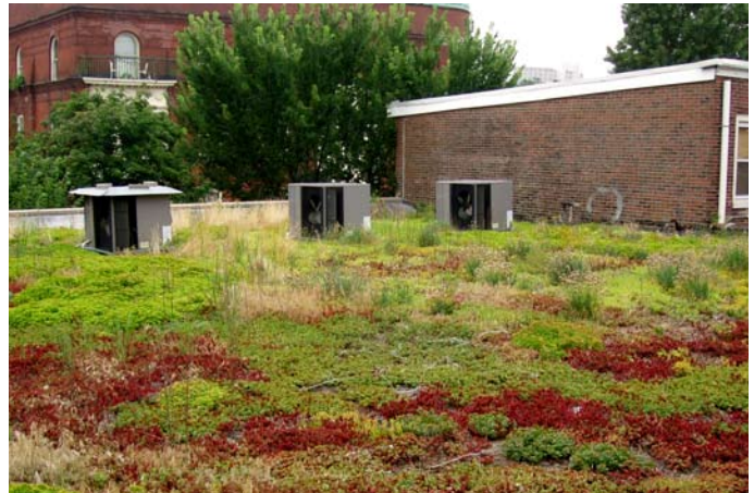
Figure 32. Green roofing installed to reduce runoff from a commercial building. Source: © Roofscapes, Inc., used by permission; all rights reserved.
