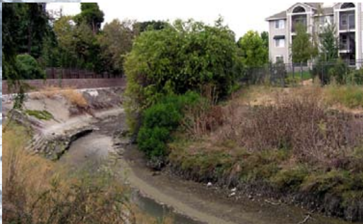
Figure 10. This section of San Francisquito Creek has been hardened and a flood wall erected to protect streamside property on the left side of the photo. Riparian vegetation has been cleared along the right side to maintain channel capacity. Photo: R. Harris.
