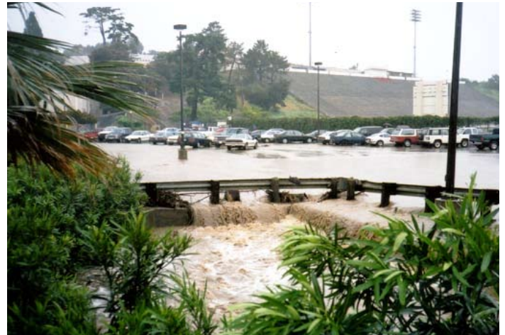
Figure 14. Storm water flowing off this parking lot carries pollutants to Honda Creek in Santa Barbara in April 2000. Photo: L. Thompson.
