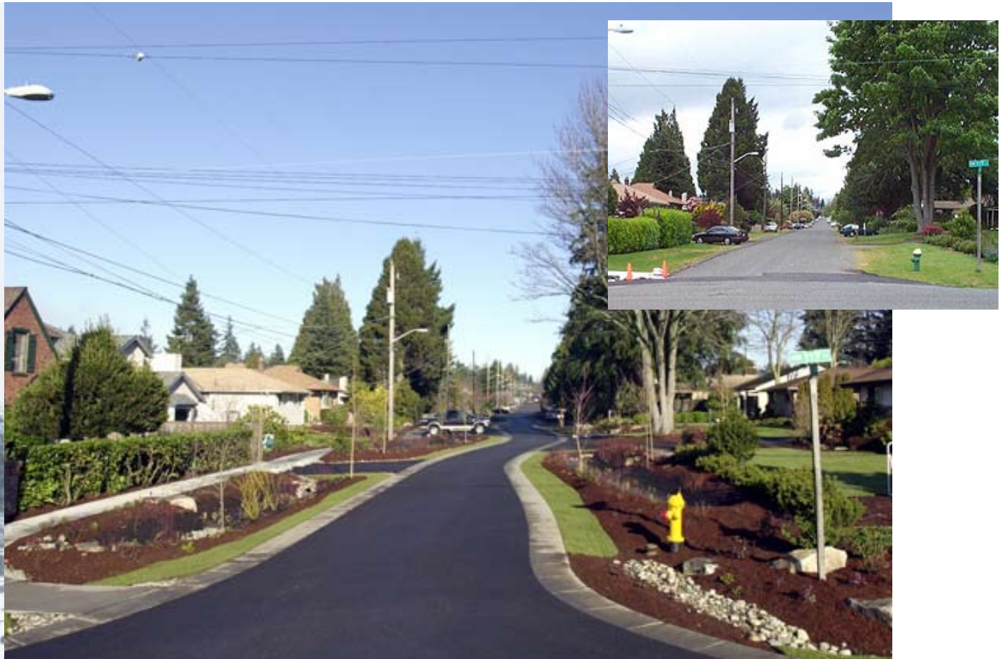
Figure 29. Seattle's Street Edge Alternatives project involved calming traffic by narrowing and curving the roadway and installing storm water retention swales. (Inset: street before the project.) Source: © 2005, Seattle Public Utilities, used with permission.
