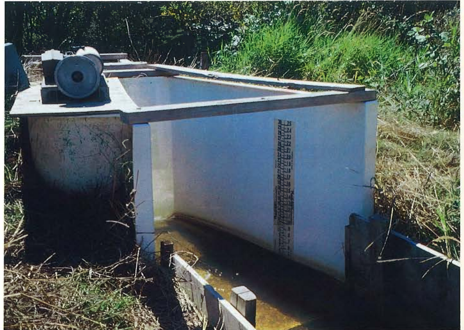
Photos 30 and 31. Ditch boxes control water flow for flood irrigation.
