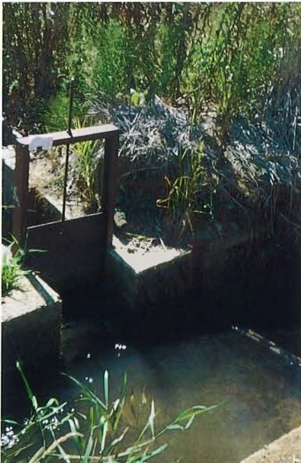
Photos 30 and 31. Ditch boxes control water flow for flood irrigation.
