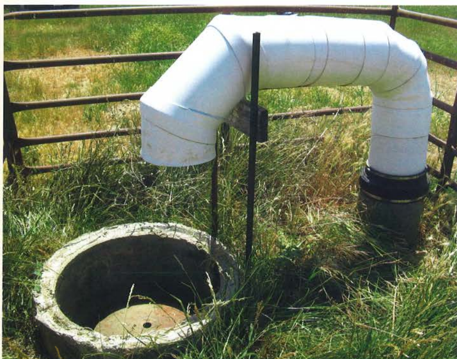
Photo 29. Water pumped into pipes for flood irrigation.
