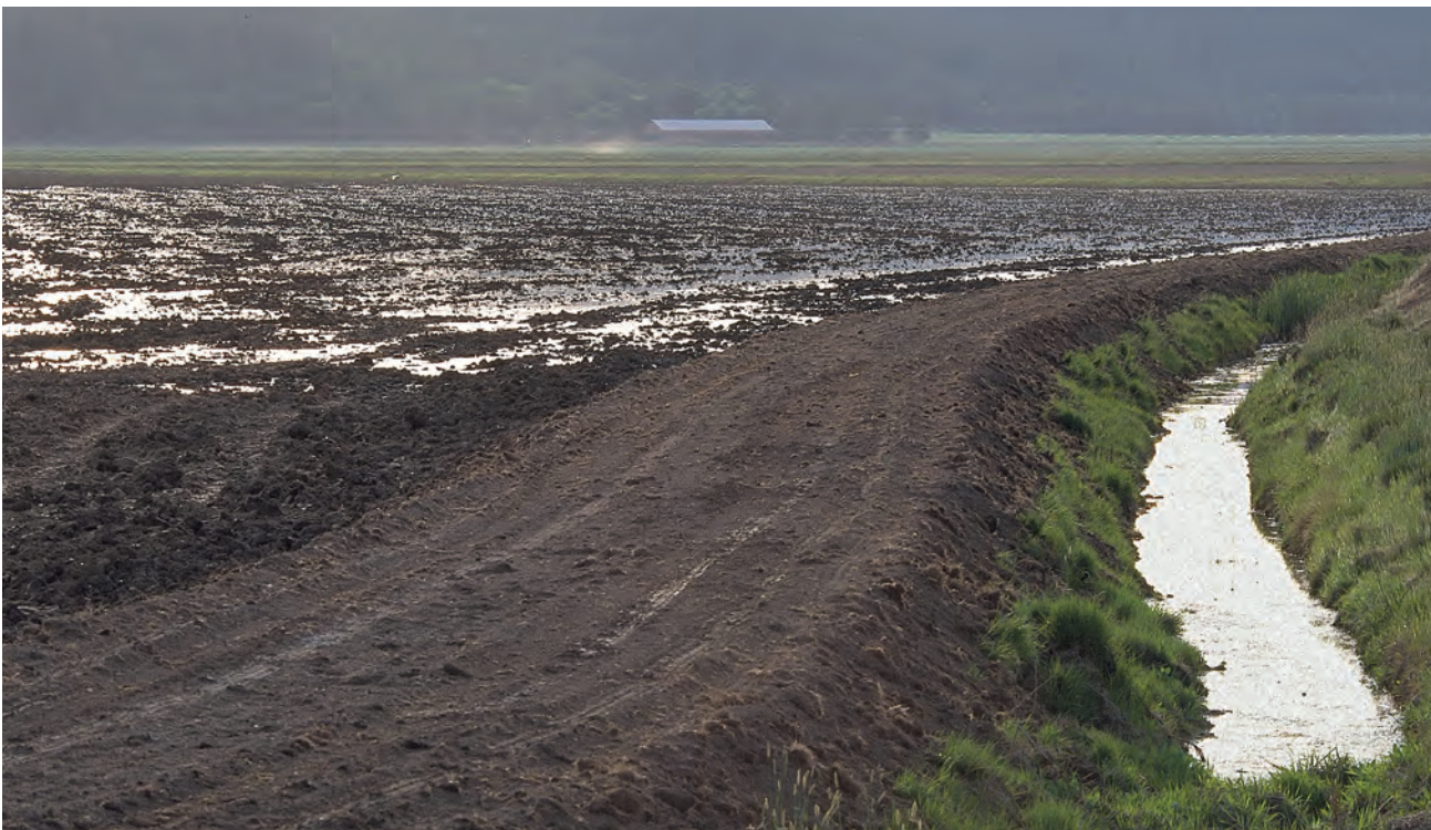
Figure 15. Wild rice levee with external drain ditch.
